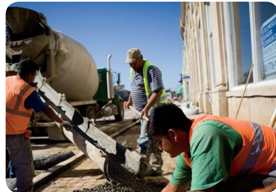
Photo: Sidewalk Construction on Liberty St.
