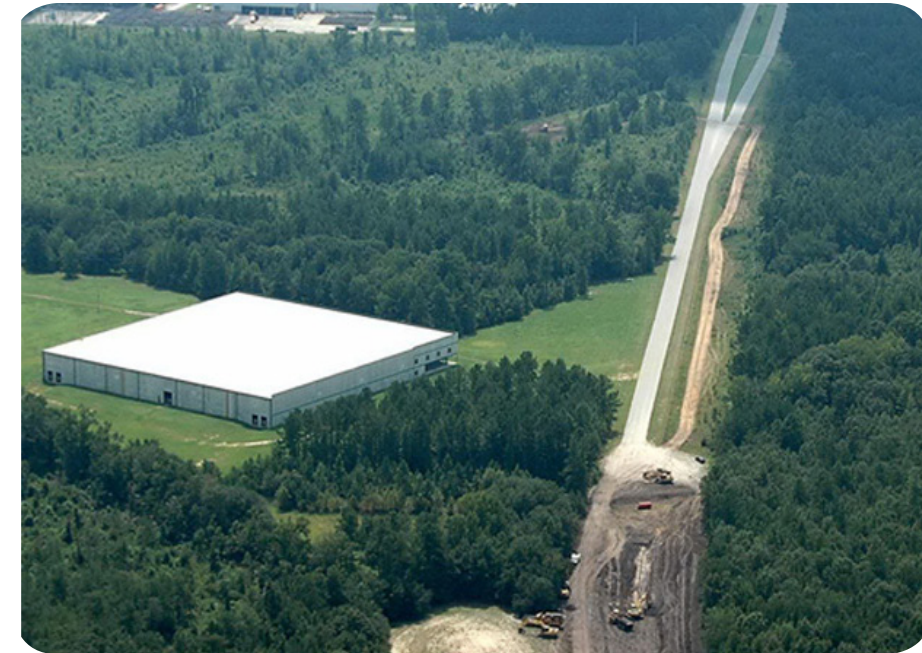
Photo: North Wise Dr. Road Construction
