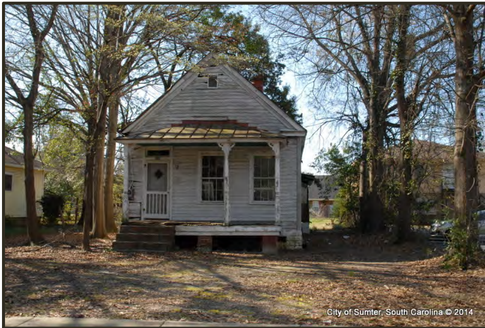
Photograph 22 Hampton Park Example of "Hazard" Condition Property
