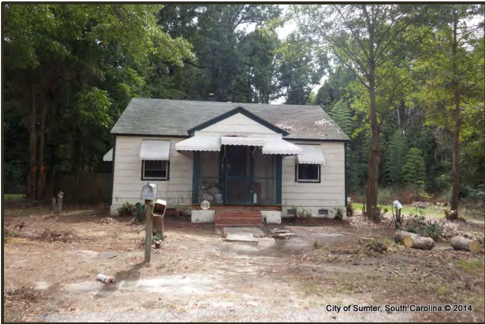
Photograph 54 Second Mill Example of "Fair" Condition Property
