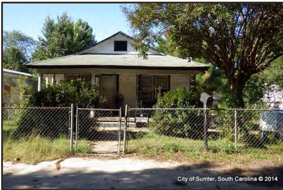
Photograph 74 Wilder Example of "Fair" Condition Property
