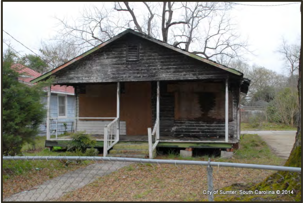
Photograph 8 Birnie Example of "Hazard" Condition Property
