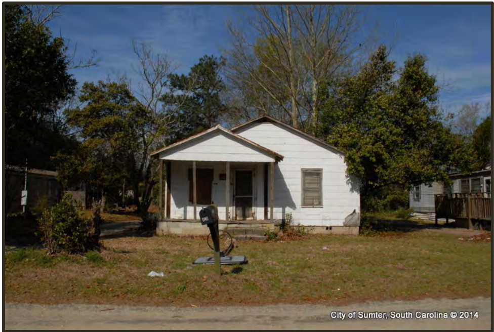
Photograph 43 Mulberry Example of "Poor" Condition Property
