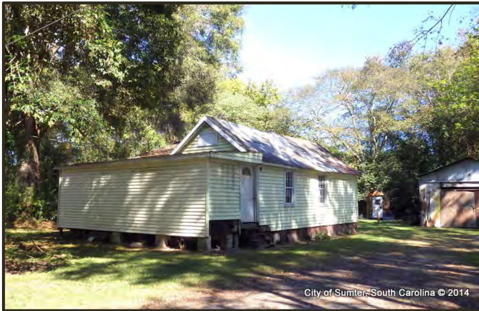
Photograph 25 Lemira Example of "Poor" Condition Property
