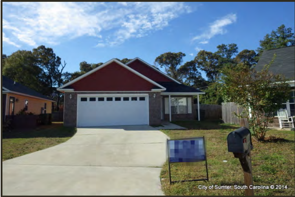
Photograph 61 Spectrum Example of "Good" Condition Property
