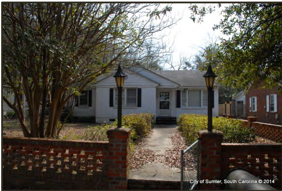
Photograph 38 Morris College Example of "Fair" Condition Property
