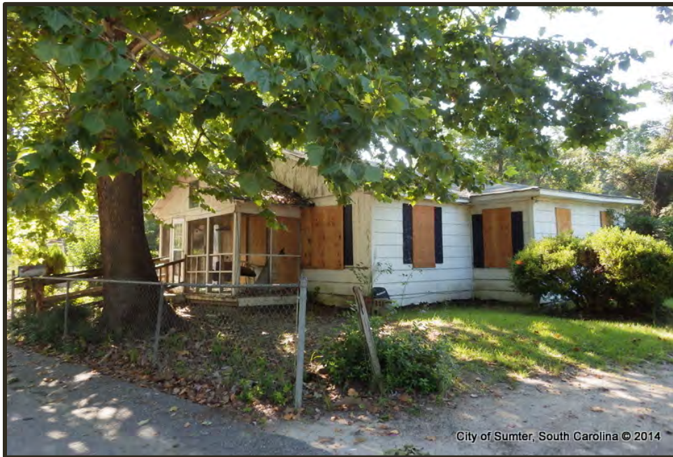
Photograph 13 Crosswell Example of "Poor" Condition Property
