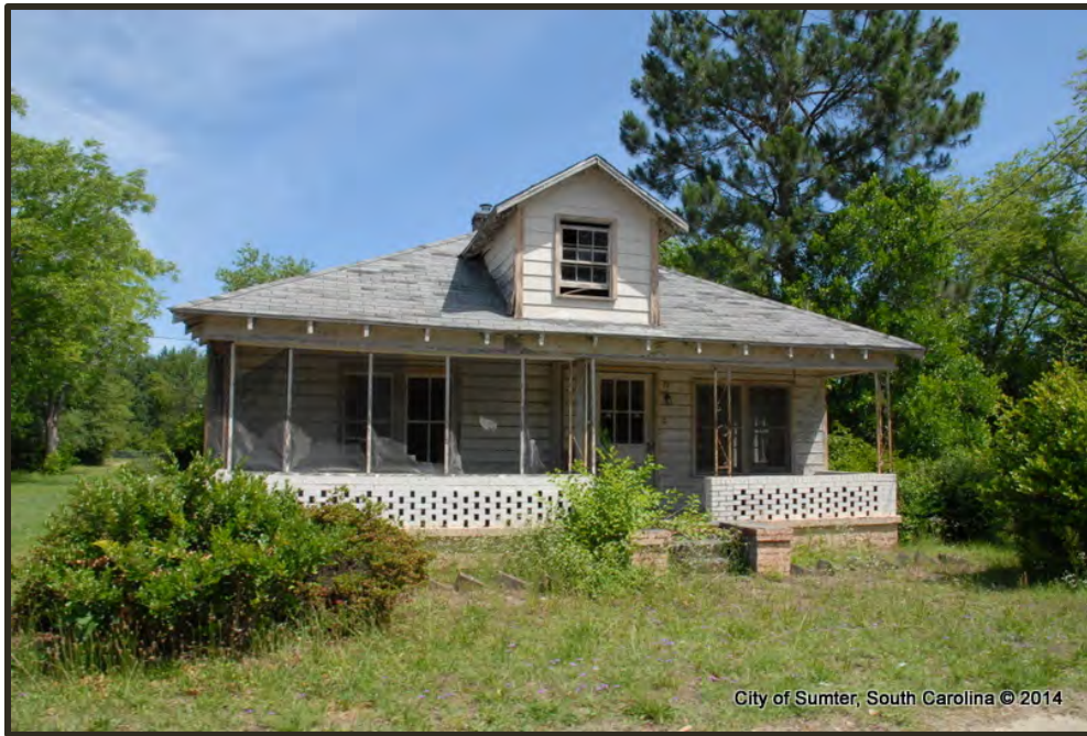
Photograph 63 Spectrum Example of "Poor" Condition Property
