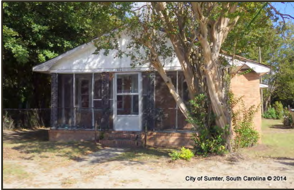
Photograph 65 Stone Hill Example of "Good" Condition Property
