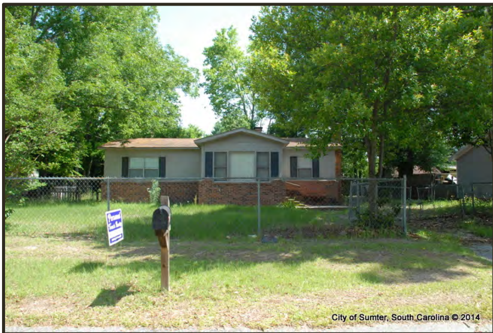
Photograph 66 Stone Hill Example of "Fair" Condition Property
