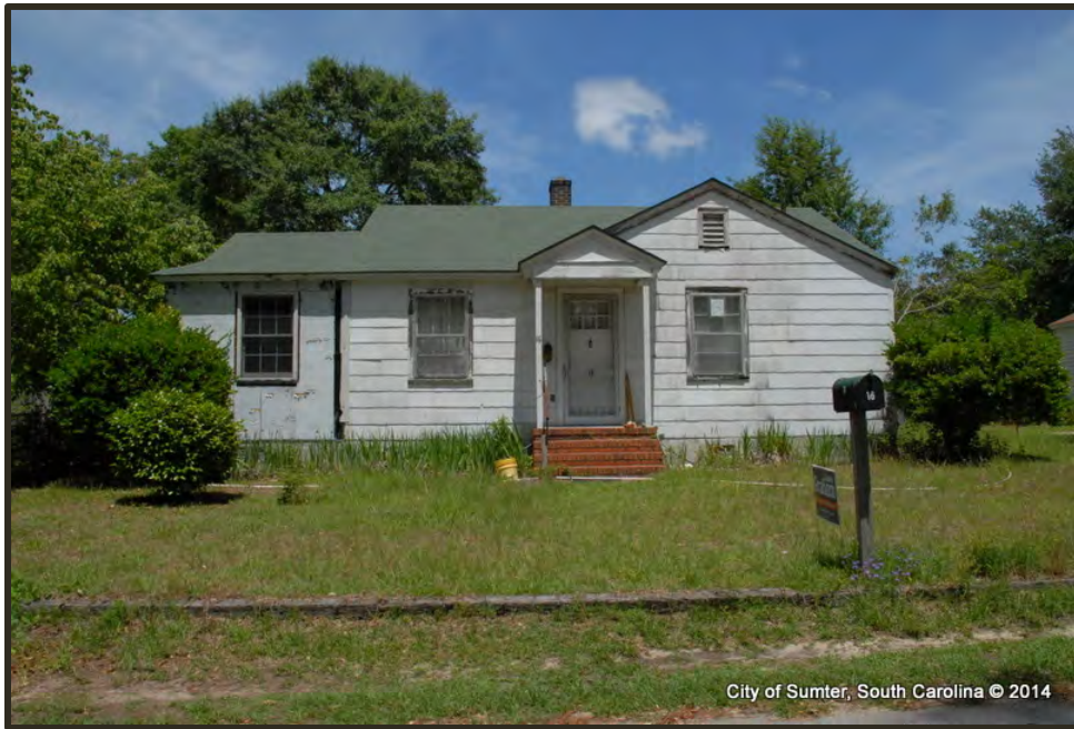
Photograph 55 Second Mill Example of "Poor" Condition Property
