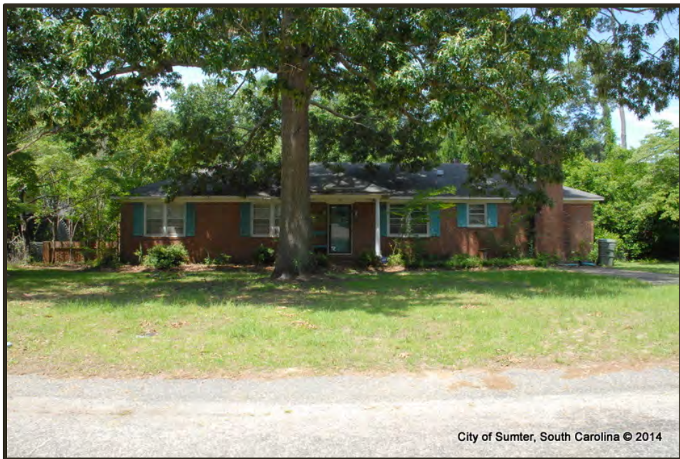
Photograph 36 Millwood Example of "Fair" Condition Property
