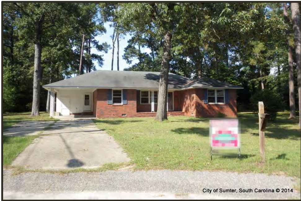
Photograph 35 Millwood Example of "Good" Condition Property
