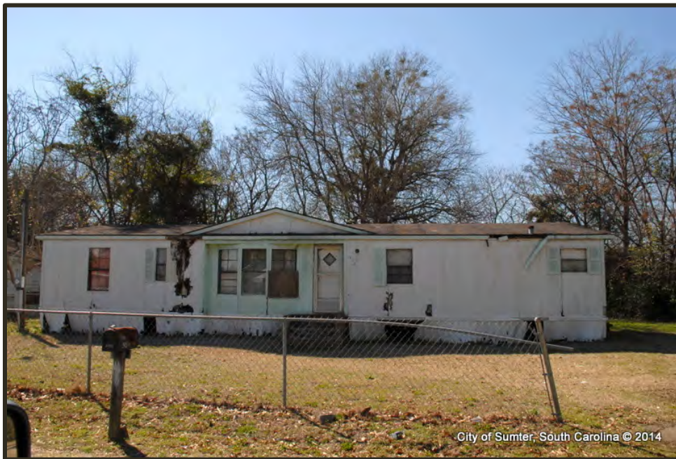
Photograph 68 Stone Hill Example of "Hazard" Condition Property
