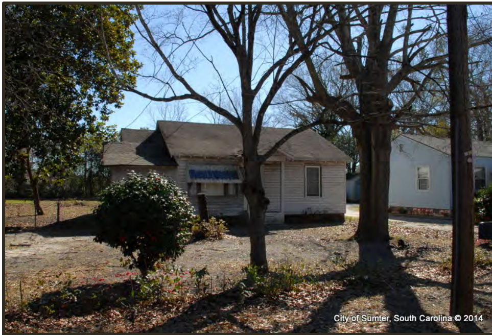
Photograph 39 Morris College Example of "Poor" Condition Property
