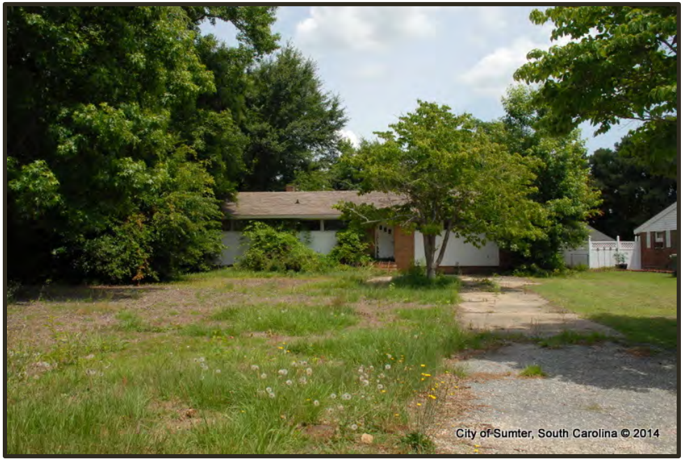
Photograph 47 Palmetto Example of "Poor" Condition Property
