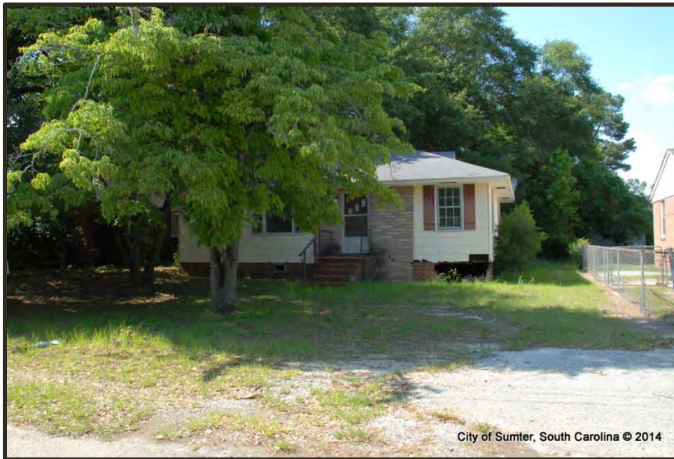
Photograph 60 South Liberty Example of "Hazard" Condition Property
