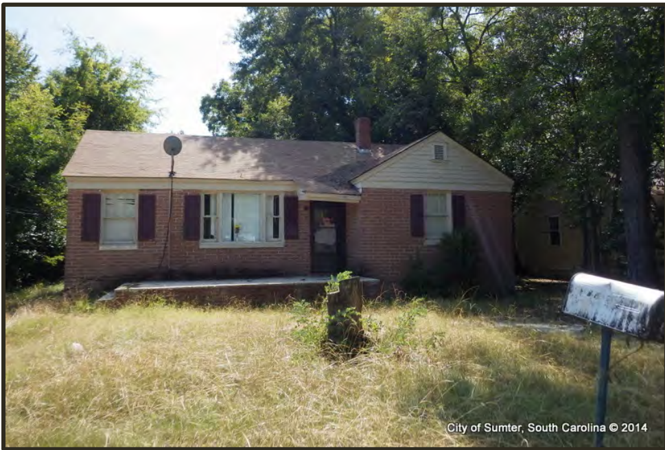
Photograph 16 Folsom Park Example of "Fair" Condition Property
