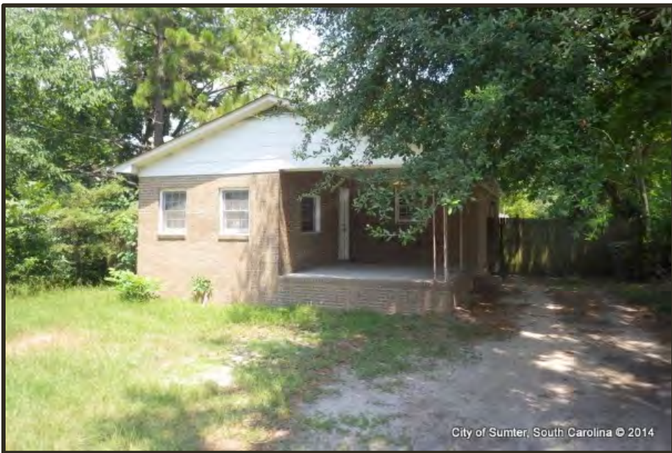
Photograph 2 Bates Example of “Fair” Condition Property
