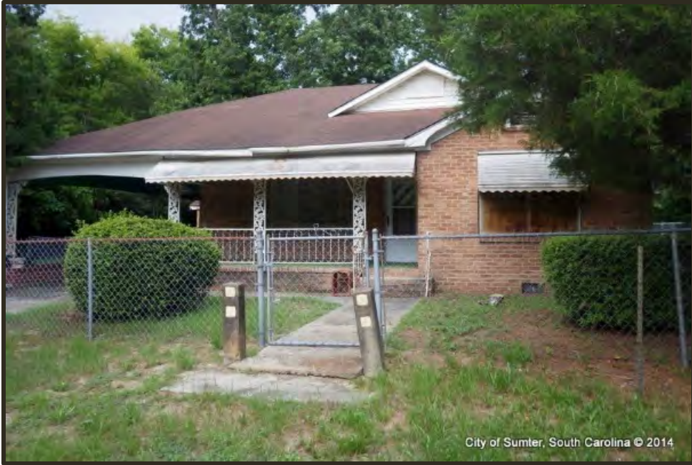
Photograph 1 Bates Example of “Good” Condition Property
