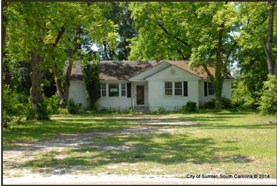
Photograph 37 Morris College Example of "Good" Condition Property
