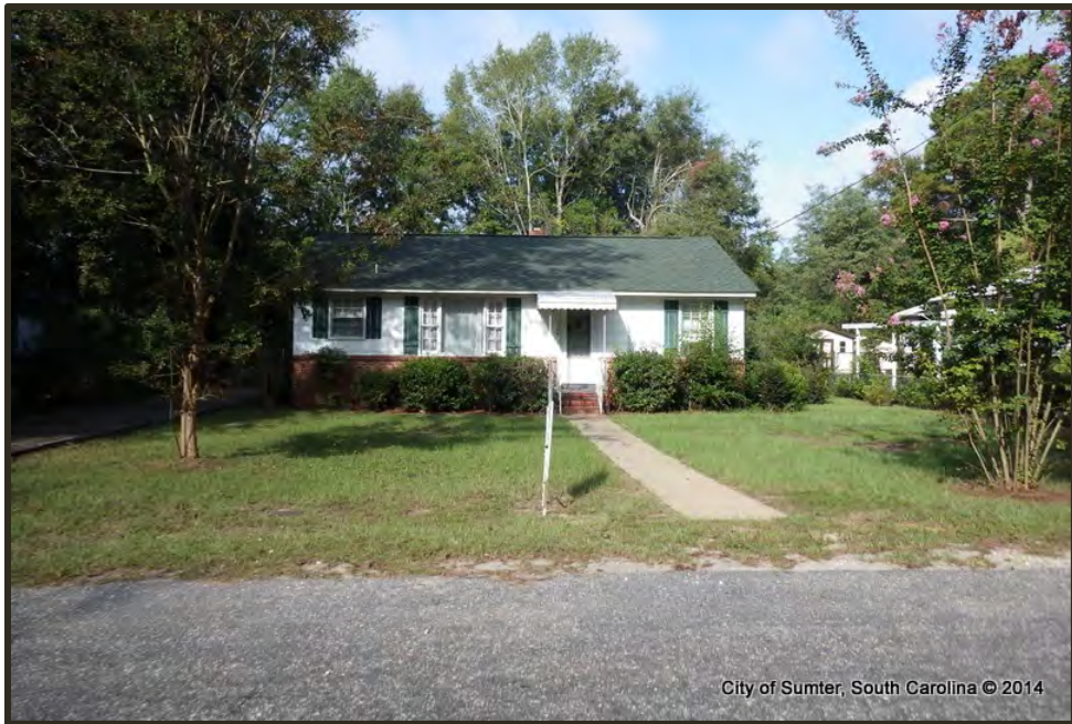
Photograph 57 South Liberty Example of "Good" Condition Property
