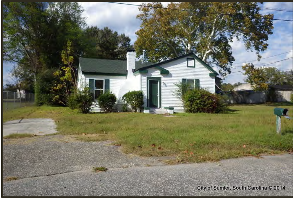
Photograph 31 Magnolia-Harmony Example of "Good" Condition Property
