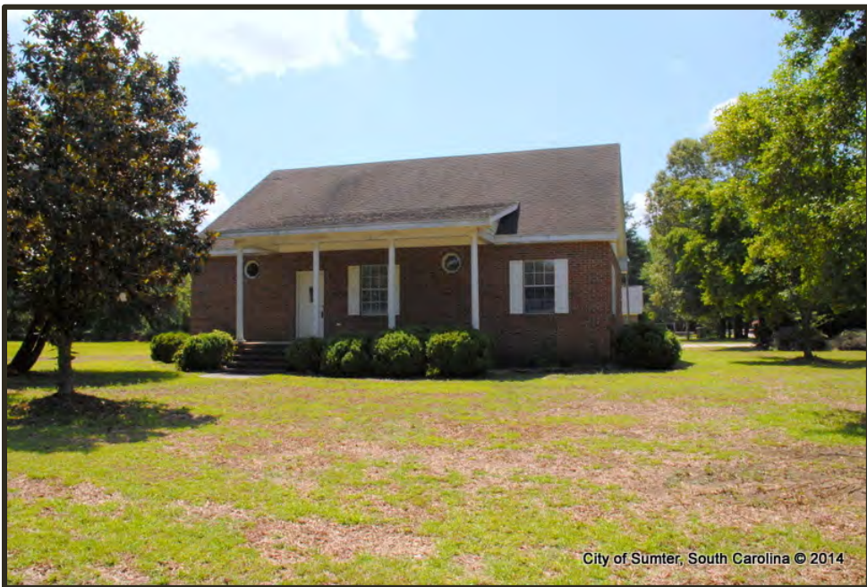
Photograph 62 Spectrum Example of "Fair" Condition Property
