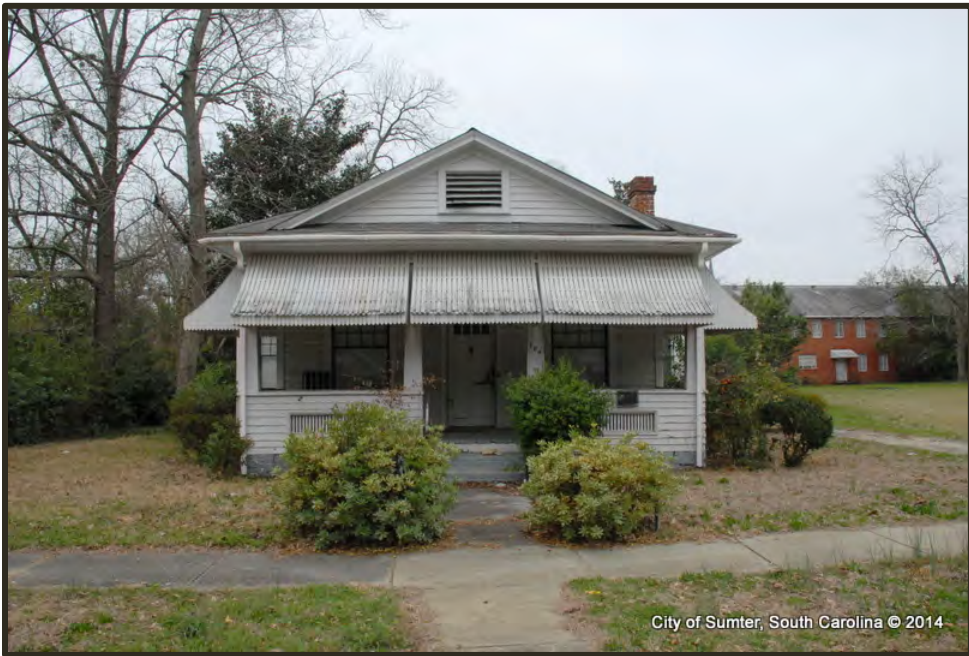
Photograph 6 Birnie Example of "Fair" Condition Property
