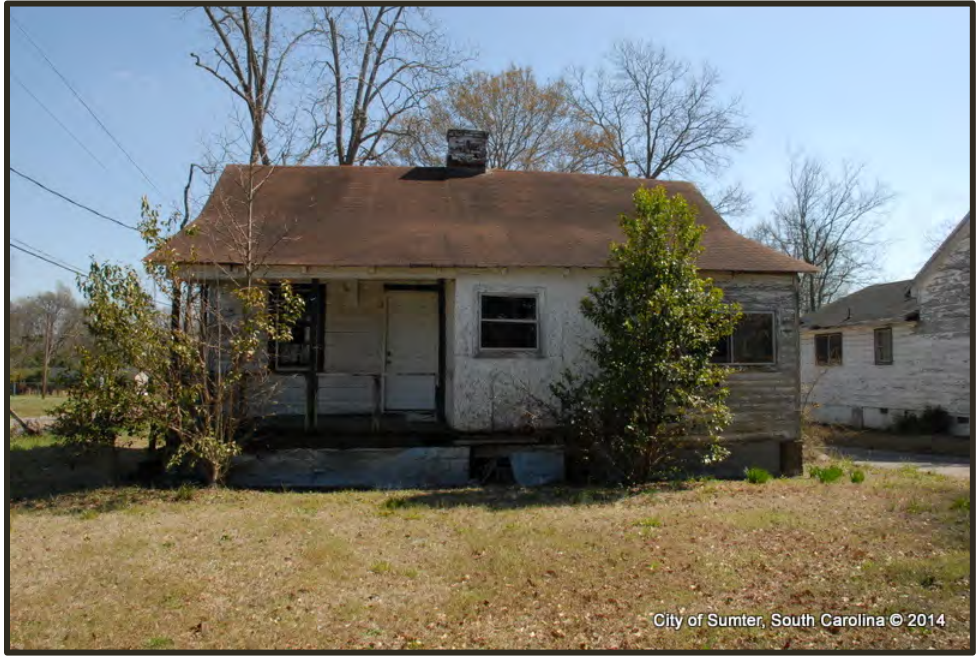
Photograph 34 Magnolia-Harmony Example of "Hazard" Condition Property
