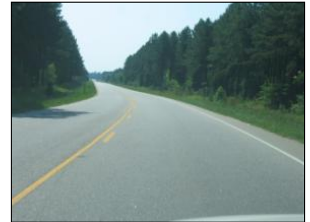
Paved Shoulder on Patriot Parkway
