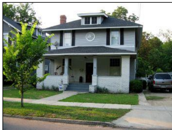
Off-Base Housing near West Hampton Avenue
