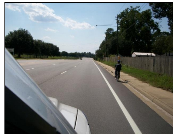
McCrays Mill Road Bicycle Lane
