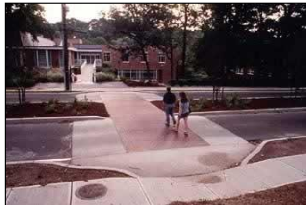
Raised sidewalk slows speeds and improves pedestrian safety (Source: www.pedbikeimages.org)
