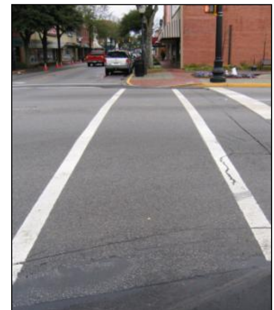
Crosswalk and curb ramp in Downtown Sumter
