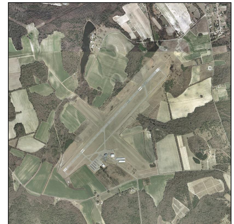
Sumter Airport Aerial
