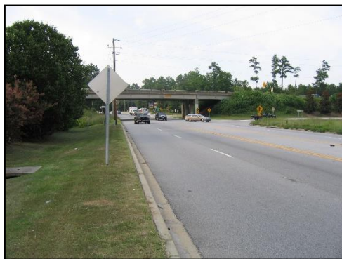
Major Arterial – Broad Street
