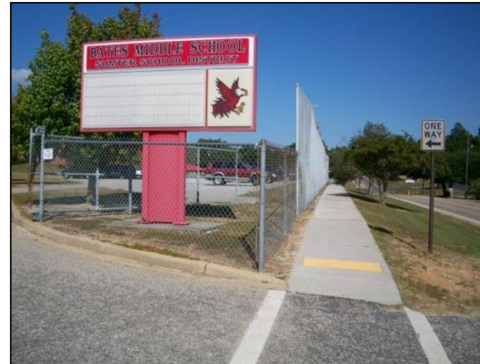
Part of the newly constructed sidewalk that connects Bates Middle School with the surrounding neighborhood.
