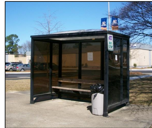
Transit stop treatment (Source: City of Sumter, SC)
