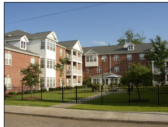
Dugan Street between Sumter Street and Main Street
