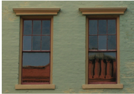
Double-Hung Sash with Decorative Lintel
