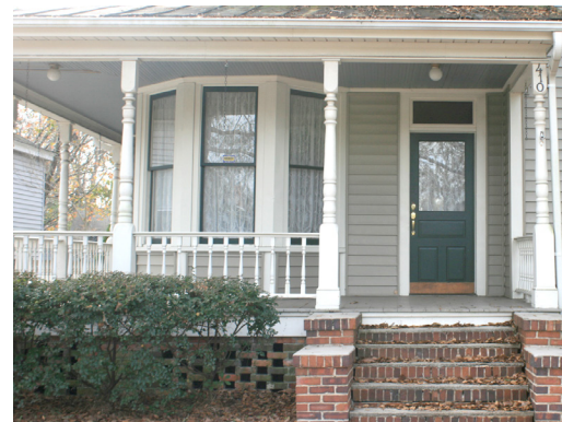
These simple, unobtrusive light fixtures are mounted to the porch ceiling.
