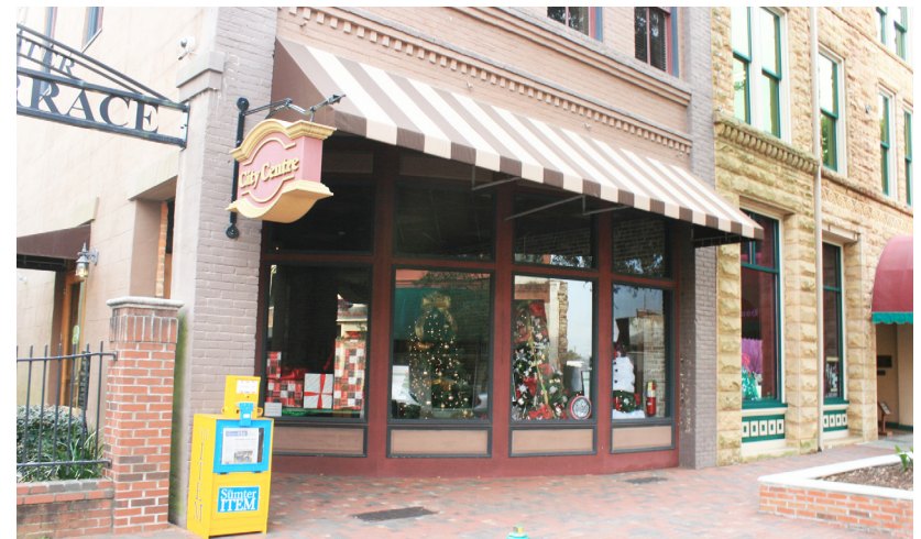
The transom and bulkheads of this storefront are simple in design and are based on the scale, proportions, materials, and colors of other commercial buildings in the district.
