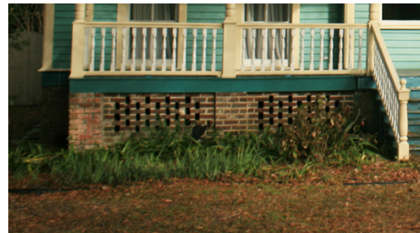
Recessed pierced brick lattice retains the visual qualities of the brick pier foundation.
