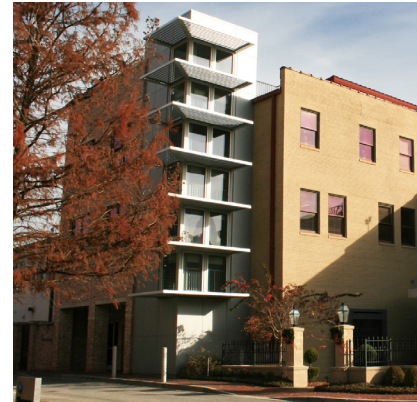
Located on the rear elevation, this addition is contemporary in design to distinguish it from the original building.
