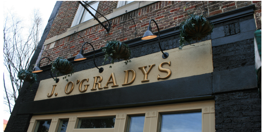
This sign is illuminated indirectly with a shielded light source.
