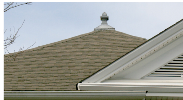
This historic roof finial was reinstalled after roof replacement.
