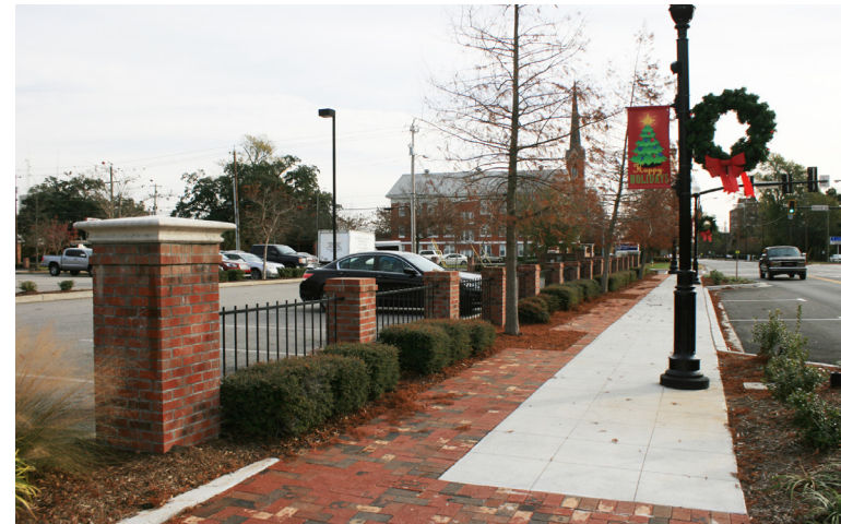
Brick piers and metal fencing continue the setback and rhythm of the downtown streetscape.
